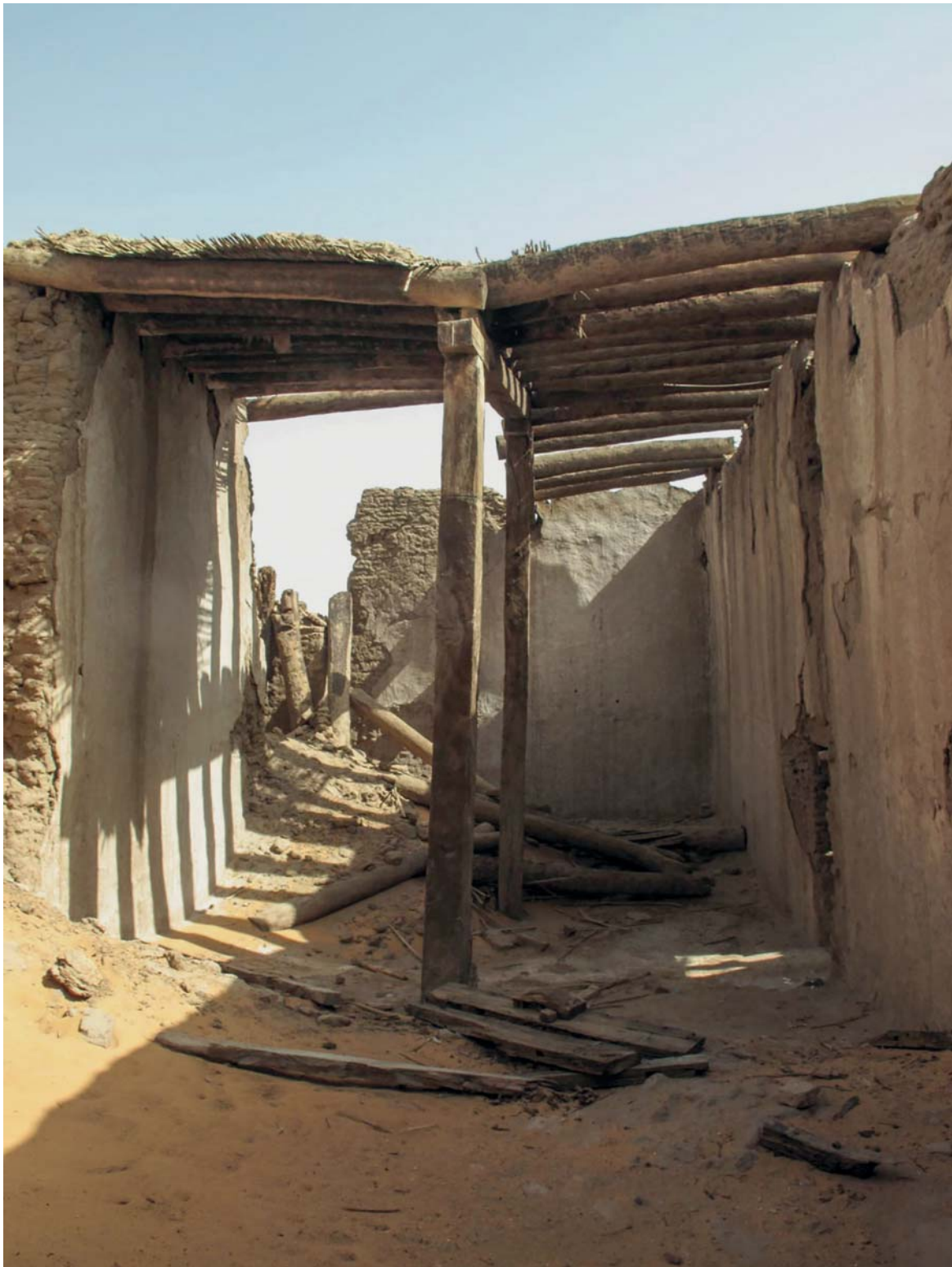
Fig. 225. Wooden posts supporting a roof in one of the houses of the Abandoned Village
