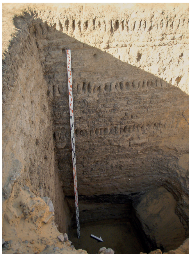
Figure 1.20. The curtain wall in Banganarti built with mud brick (photo Mariusz Drzewiecki)
