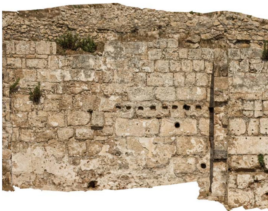
Fig. 2-10. East wall of Basilica Q, a close-up of its northern stretch; note the series of horizontal sockets presumably for the gallery supports, and the interrupted courses of the masonry to the left of it
