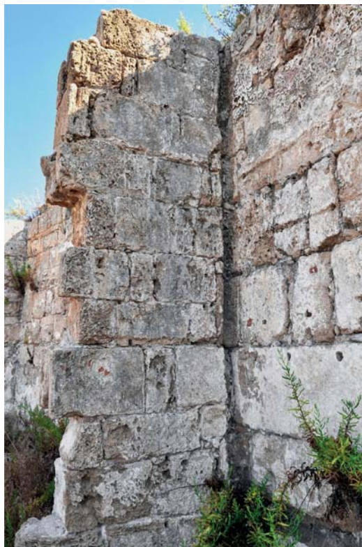
Fig. 2-9. Partition wall between the presbytery and the northern aisle; note that it is not engaged with the east wall
