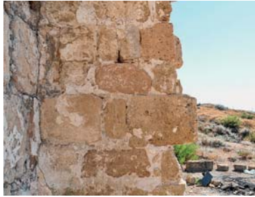
Fig. 3-5. Type 2 mortar spread over the joints of the wall separating the northern aisle from the nave of the basilica
